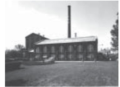
Atlanta Waterworks Hemphill Pumping State c1950
