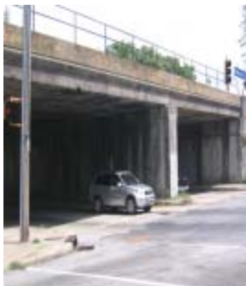
Ralph David Abernathy Overpass
