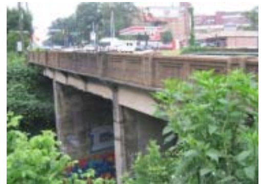
Peachtree Road Overpass
