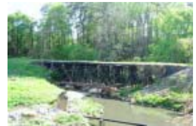
Wood trestle over Clear Creek behind Ansley Mall
