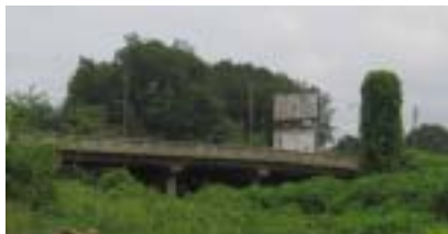
Edgewood Avenue Overpass
