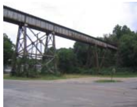
North Avenue Overpass
