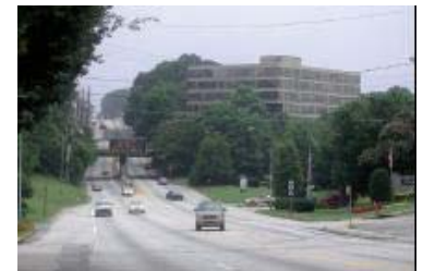
Northside Drive Overpass
