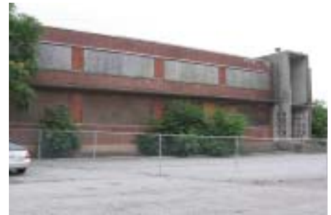
Truck transfer facility, University Avenue
