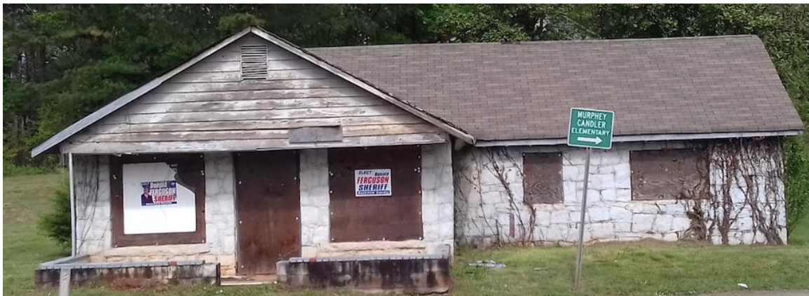
Commercial building at corner of Browns Mill Road and Klondike Road. Example of a Cross-Gabled Roof.
