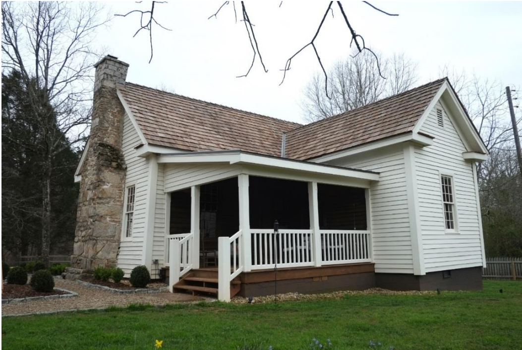
7241 South Goddard Road (ca. 1850) – Housworth-Moseley House – granite is used in chimney construction.
