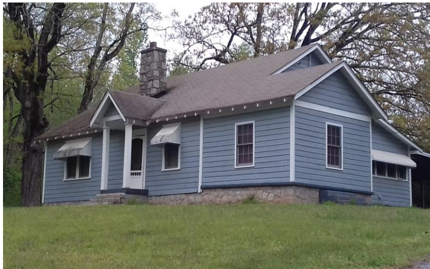
7126 South Goddard Road. Example of a granite chimney.
