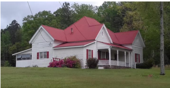
4357 Klondike Road. Example of appropriate siding.
