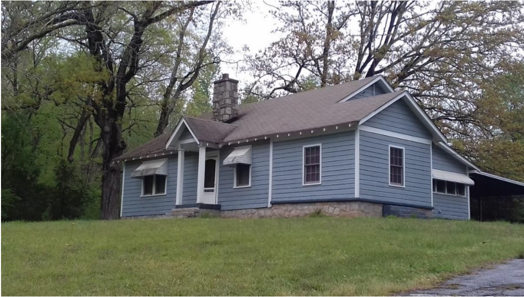
7126 South Goddard Road (ca. 1939) – granite used on foundation, chimney and steps – Craftsman style exposed rafters, bracket on gable end and square columns supporting roof over the stoop.
