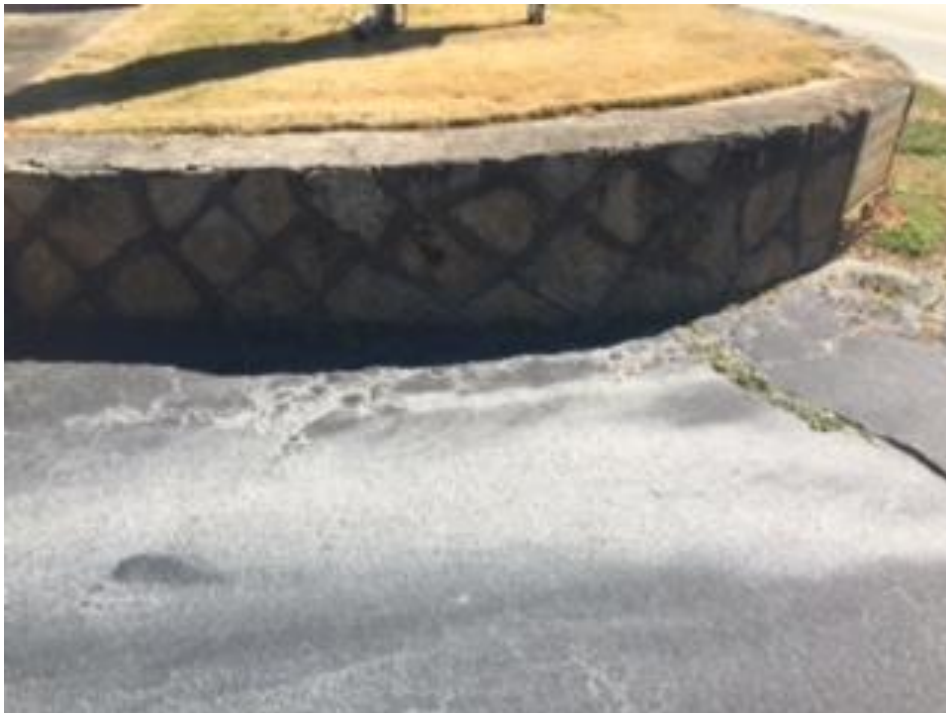
Example of granite retaining wall.
