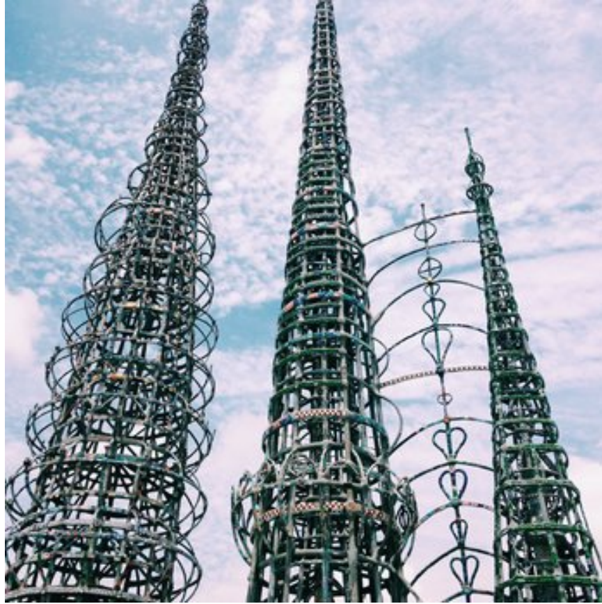
Figure 4.22 Simon Rodia's Watts Towers
