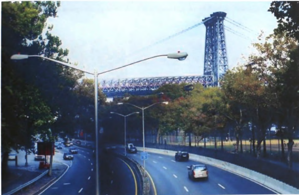
Figure 51: Current picture of FDR Drive, north of Corlears Hook
