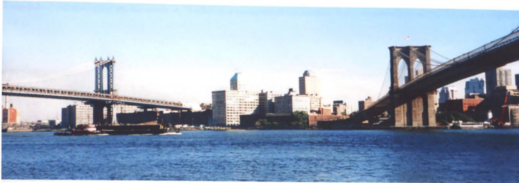
Figure 58: View of Brooklyn from the Lower East Side, between Manhattan and Brooklyn Bridges.
