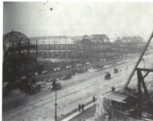
Figure 7: Photo of Chelsea Piers construction.
