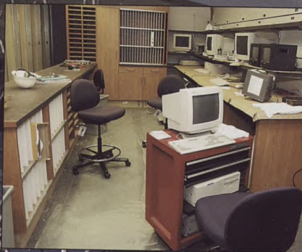
Under construction. Clinical staff will use computers in this area to monitor patients who are undergoing radiotherapy in one of the linear accelerator rooms.
