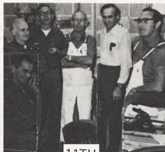
11TH MAINTENANCE, MECHANICAL SHOPS
