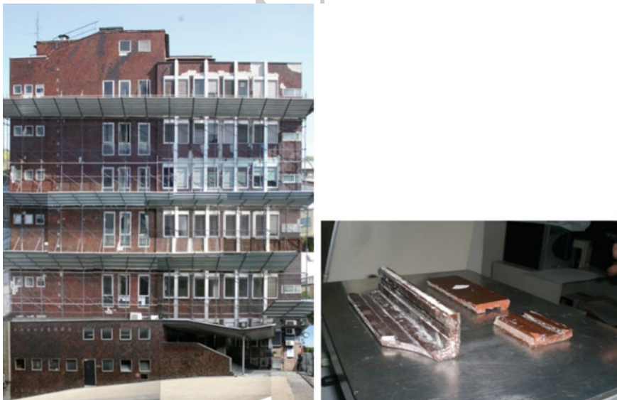
Fig. 3 Building 12 in Campus Leonardo (left); details of the tiles of Building 12 (right)
