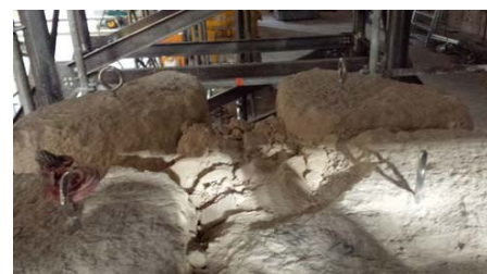
Figure 8. Top images of a pillar during disassembly; in the centre, the irregular mortar core of the column
