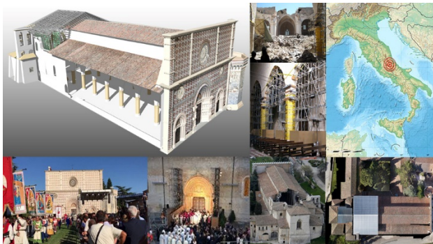
Figure 1. Earthquake damages, the Holy Door during the Jubilee Forgiveness procession, and 3D textured models
