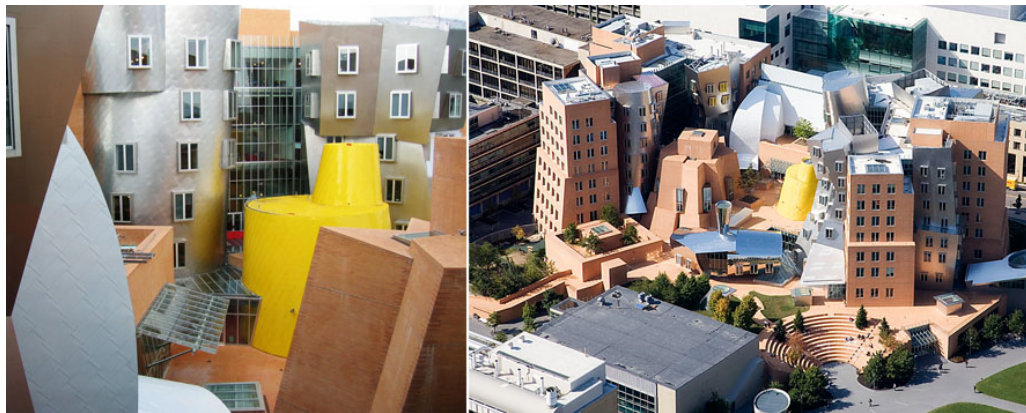
Figura 2.2.9 Stata Center del Massachusetts Institute of Technology , Cambridge, Massachusetts. Gehry (concluido en 2004)
