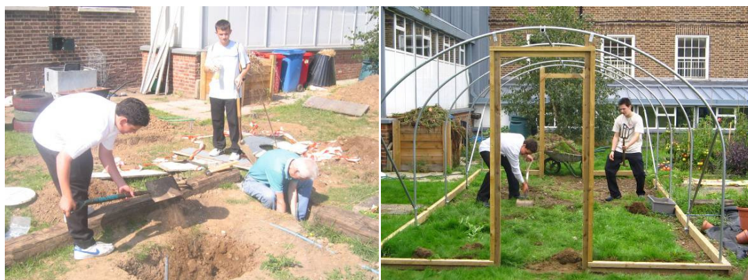
Figure 18 Students helping to build the polytunnel (Source: Glebe School)
