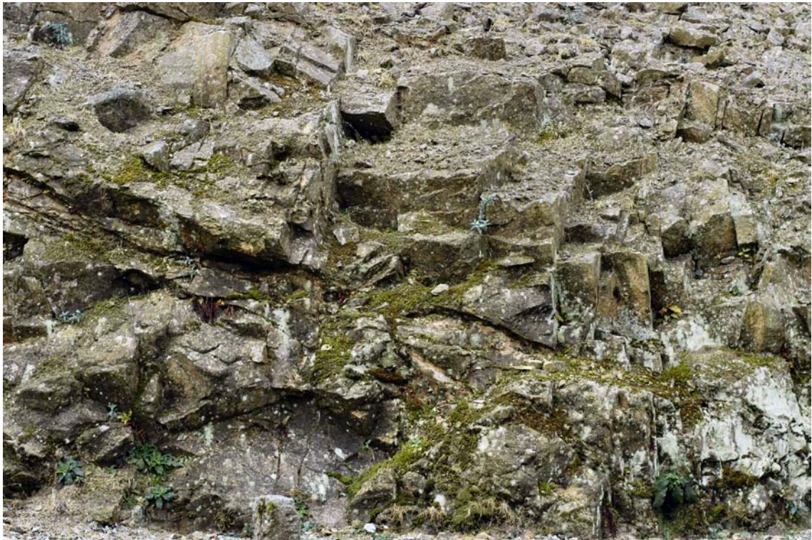
Figure 5-4. Image showing blocky nature of the granite rock mass at the Tremough Campus road cutting (3 m wide, 2.5 m high rock face, looking south).
