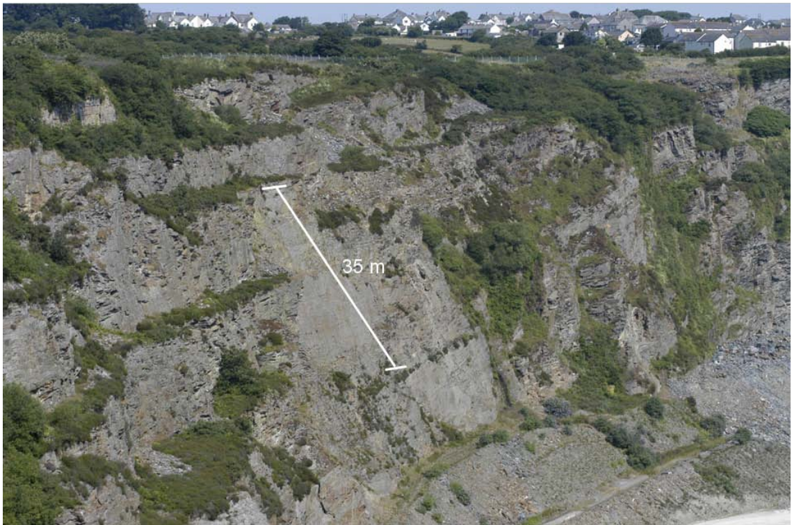
Figure 4-50. Photograph of the 1967 failure face at Delabole Quarry viewed NNW, with the town of Delabole in the background. The slope is ~100 m high from the haul road.
