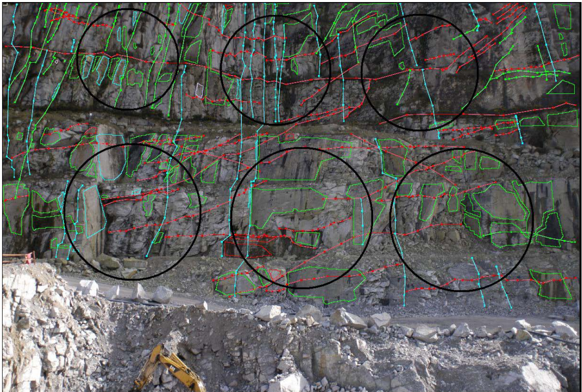
Figure 5-29. Example circular window mapping from orthoimage of Carnsew Quarry (lower circles 6 m diameter, upper circles 10 m diameter). Using an orthoimage removes the perspective bias of using normal photographs. The circles were scaled using ImageJ (Rasband, 2007) and superimposed onto the orthoimage showing the discontinuity traces coloured according to orientation.
