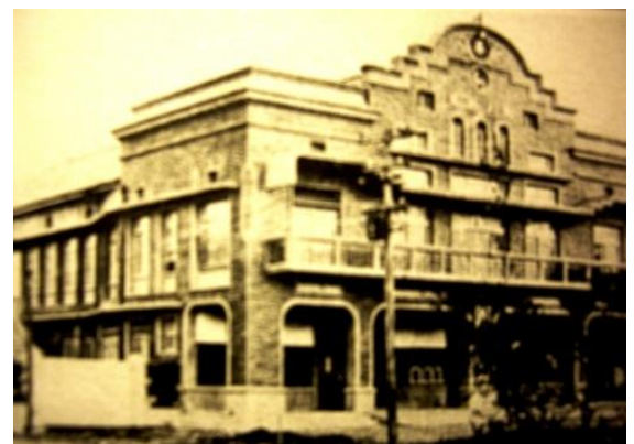
Figure 2.5 The Yunlin Theatre. It combined with Japanese and Western baroque styles (1930) (Source: Chiu, 2006)
