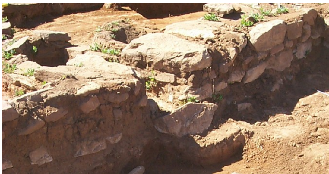
Figure 2.58. Room 33 wall vent through front wall (photo taken after subflooring). Note small vertical slab just in front of opening.
