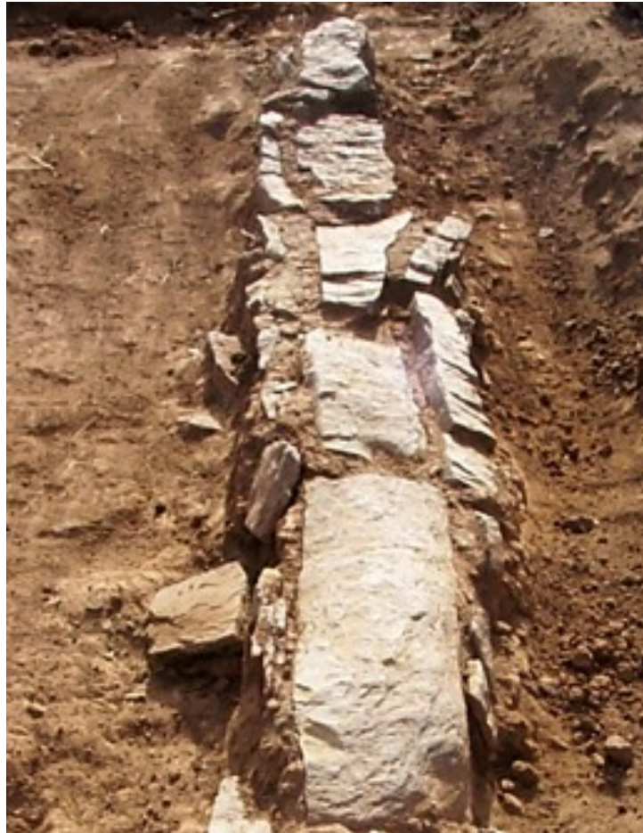
Figure 2.25. Early Pueblo II wall top showing 'veneer' on both faces to obtain desired thickness.
