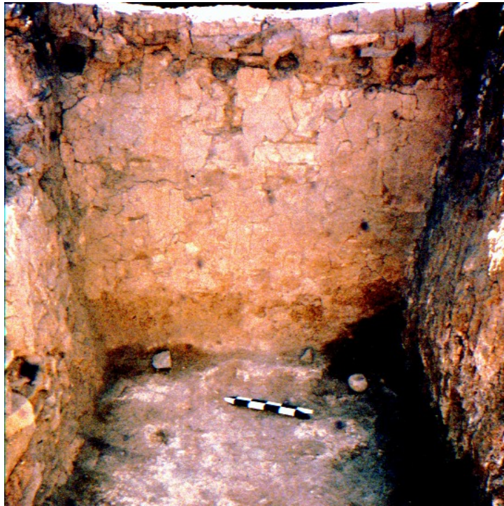
Figure 2.72. West face of the corner room wall (note plastered surface and ends of the roof beams of the corner room).
