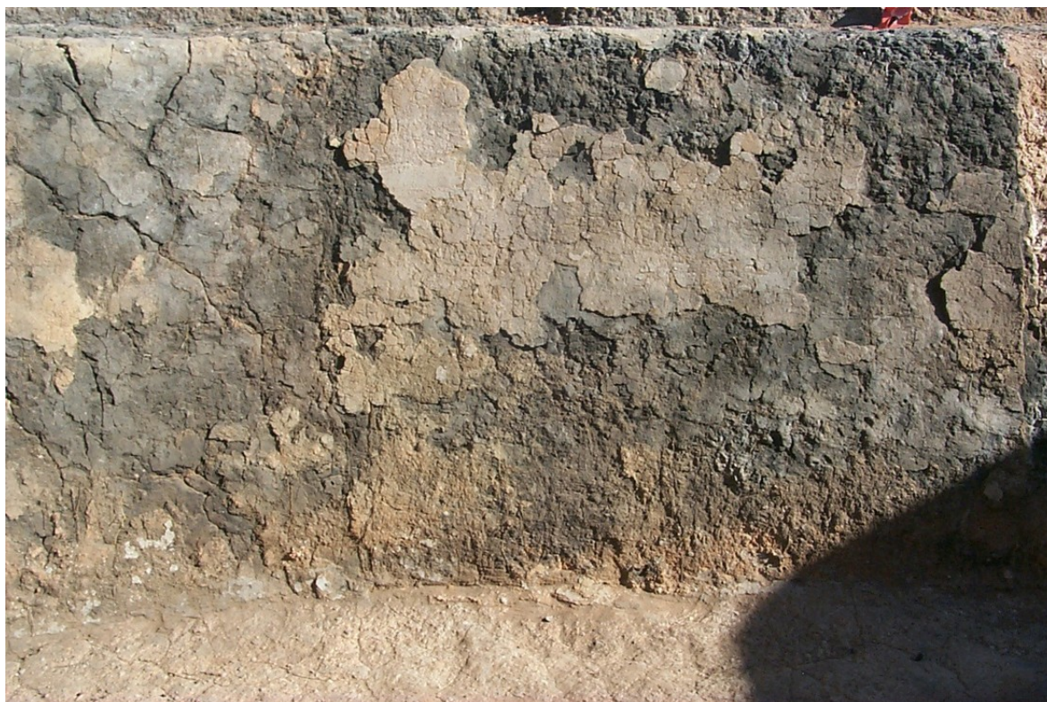
Figure 2.127. Kiva K wall plaster showing multiple layers.
