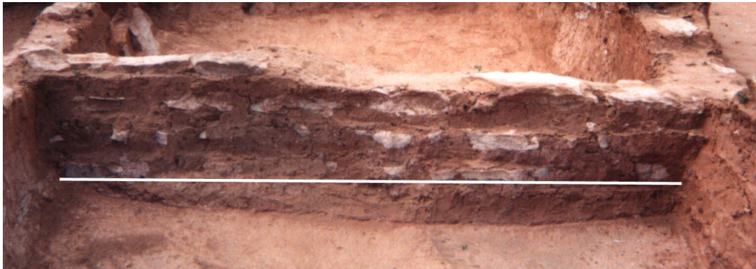
Figure 2.27. Middle Pueblo II wall showing the base of the wall (white line) above the final floor surface.
