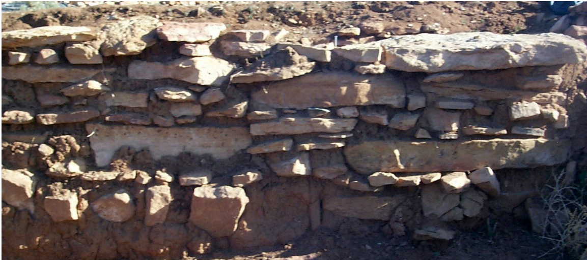
Figure 2.51. Room 30 north wall masonry, interior face.
