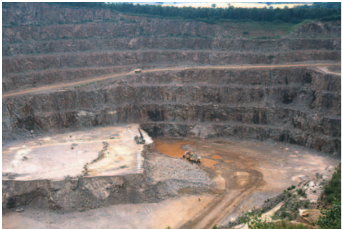
Very large active aggregate operation in Ordovician granodiorite. Mountsorrel Quarry, Leicestershire.
