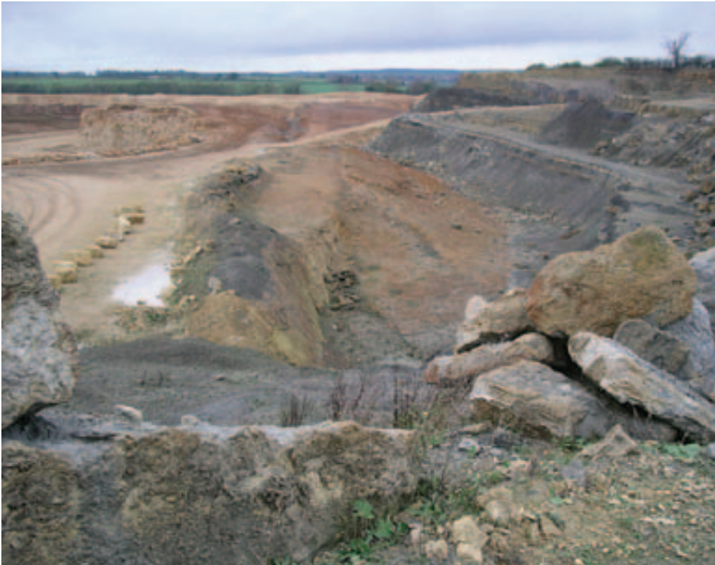
Part of a large quarry extracting cement raw materials. The quarry exposes a complete sequence of Middle Jurassic strata. The view shows Lincolnshire Limestone Formation, Rutland Formation ('Upper Estuarine Series'), Blisworth Limestone Formation, Blisworth Clay Formation, Abbotsbury Formation (Cornbrash), and Kellaways Beds (clay and sands). A large variety of fossils found at the site include ammonites, bivalves, echinoids, gastropods and rare vertebrate remains. There is minor faulting. Ketton Quarry, near Stamford, Lincolnshire.
