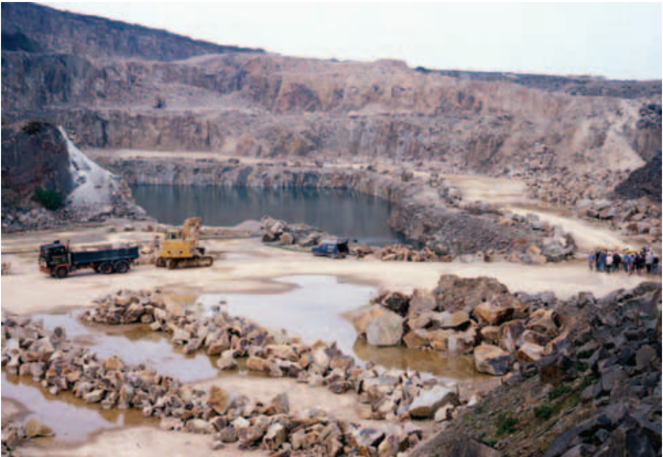
An active aggregate quarry which would present significant hazards to visitors through unstable faces and inadequate edge protection at the crests of faces. The visitors could examine the large blocks of granite in the foreground without significant risk if there were no vehicle movements. The photograph was taken prior to implementation of the Quarries Regulations, 1999.
