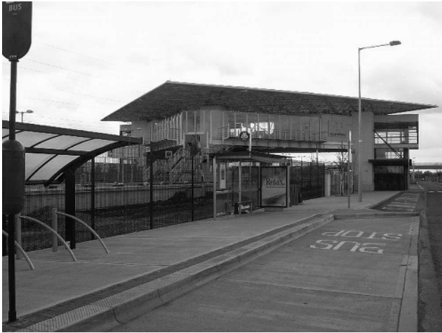
Figure 5. Adamstown central rail station (A in Figure 4)
