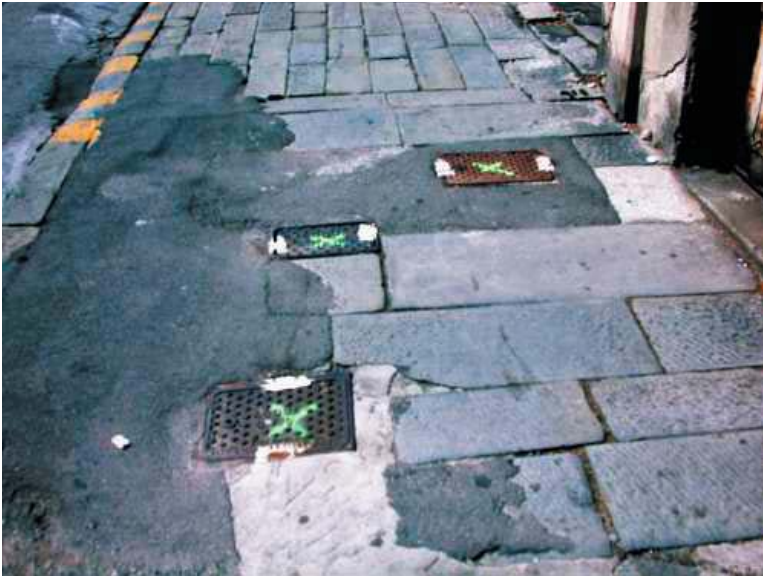
Fig.4 - Welded manholes in the red zone.
