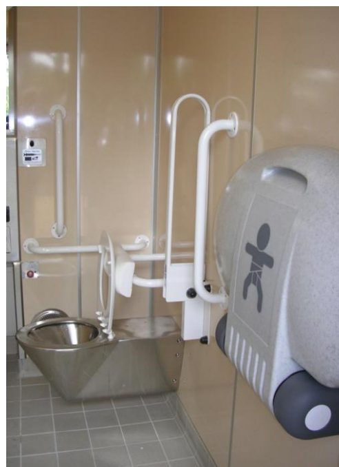
Combined accessible/baby changing facility. (Richard 2003) VivaCity 2020
