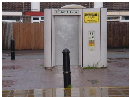
The top APC looks quite civilized but the bottom one is unattractive and uninviting. (Richard 2005) VivaCity 2020
