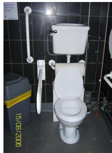
The unisex accessible cubicle. (Richard 2006) Vivacity2020
