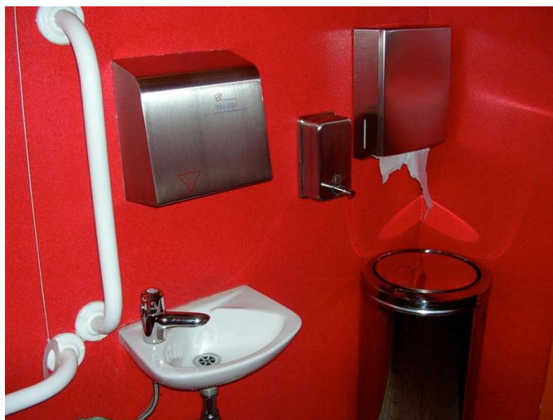
Paper towels should be provided in addition to warm air dryers. Note incorrect positioning of soap dispenser. (Bichard 2006) VivaCity 2020
