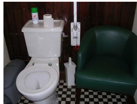
A chair has been placed in the transfer space of this accessible toilet, preventing a person who needs to side transfer onto the WC pan from accessing the space. (Bichard 2005) VivaCity 2020
