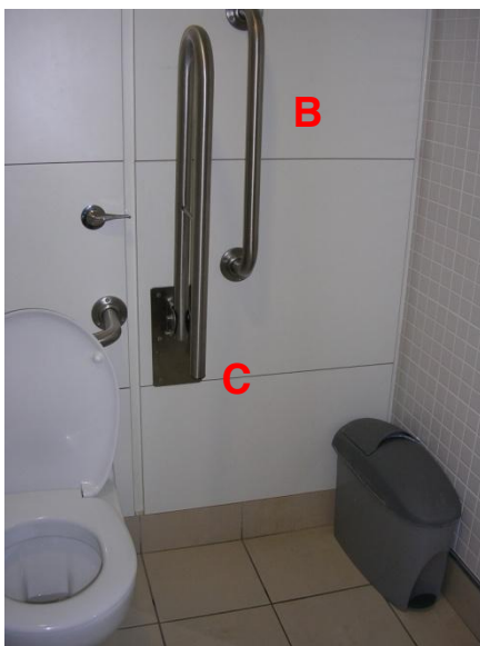
Grab rail C. Stainless steel is not the best material for this rail. (Bichard 2005) VivaCity 2020
