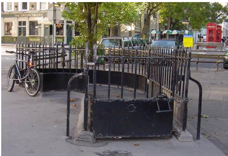
Most of Clerkenwell's Victorian subterranean provision has been closed. Clerkenwell Green Toilets. (Bichard 2003) VivaCity 2020
