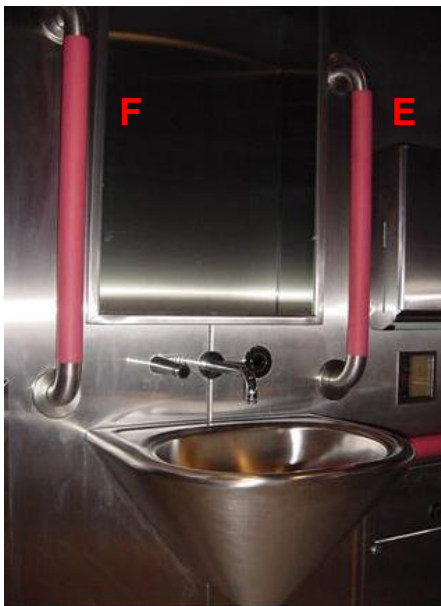
Grab rails E and F. (Bichard 2004) VivaCity 2020
