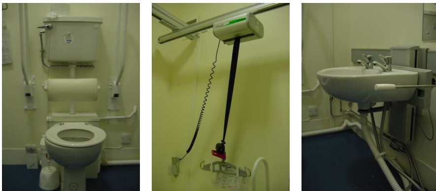
PAMIS toilet, hoist and height/space adjustable basin. (Richard 2004) VivaCity 2020
