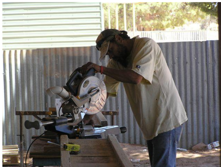
Figure 13: Locally trained tradesperson working on new housing construction at Koonibba 2007
