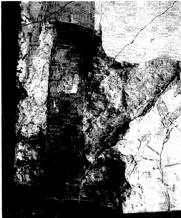
Figure 35: Post-failure condition of Cazaly Hanger (concrete removed)
