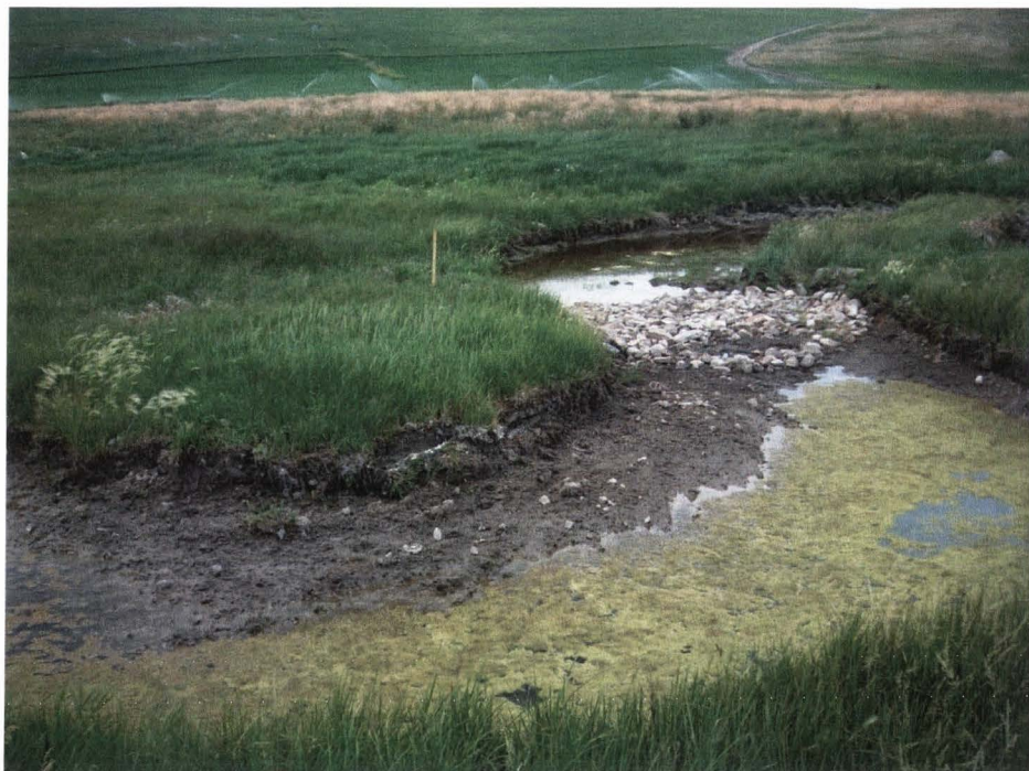
Figure 6- Inside bend of newly constructed channel within a sedge/rush community at the Trout Creek site.
