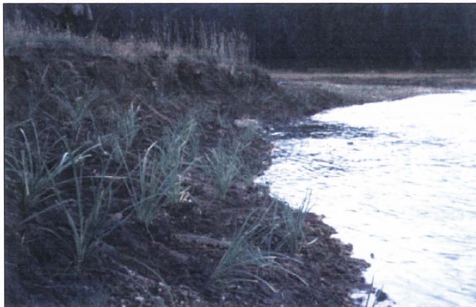
Figure 5.4. Native, water-loving small-fruited bulrush are planted into exposed soil of an outside bend in Phase I, RRRMA, Lower Red River Meadow Restoration Project.
