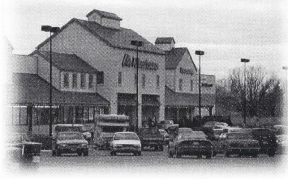
Figure 29. Albertson's Agricultural Theme Commercial Complex – Lehi, Utah
