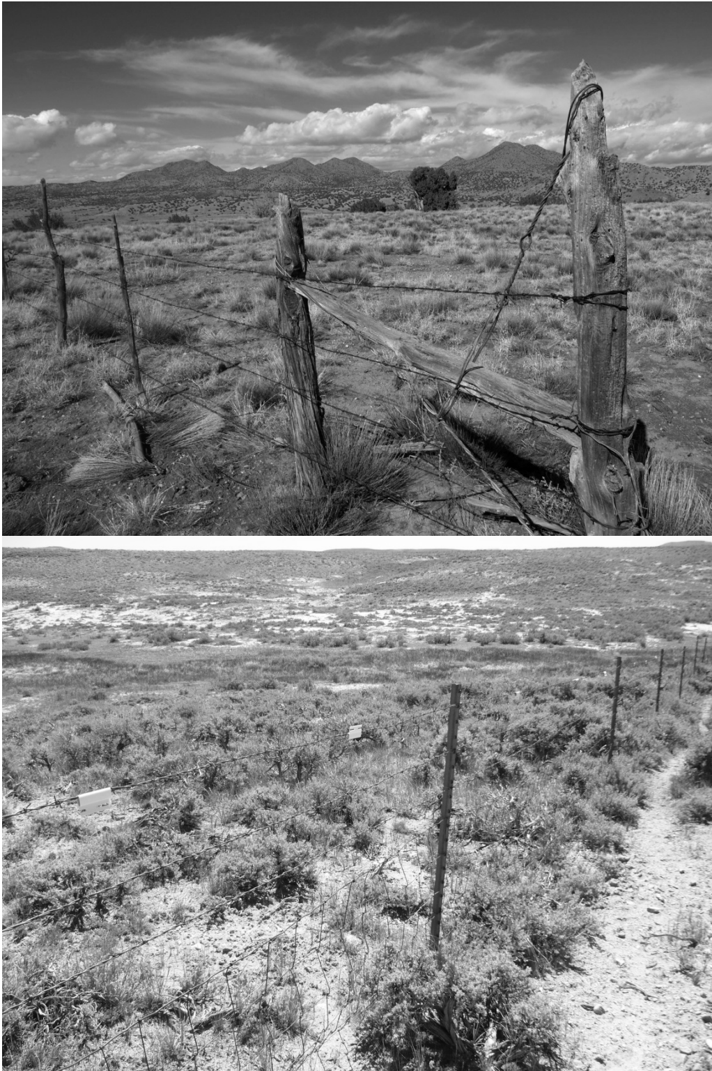
Figure 4-6. Wooden post (Upper) and metal post (Lower) fence construction types typical within the study areas.
