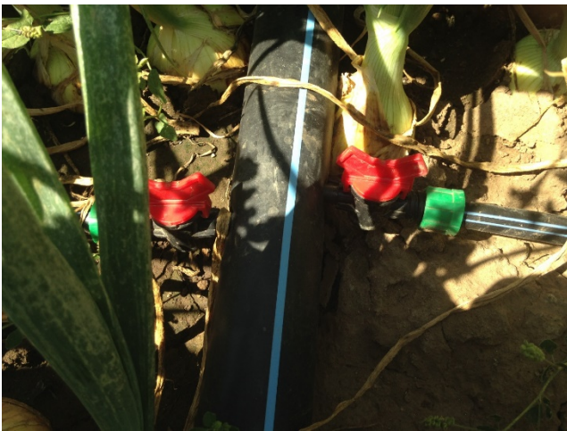
Figure 5. Flexible pvc header line with manual connectors drip tape.
