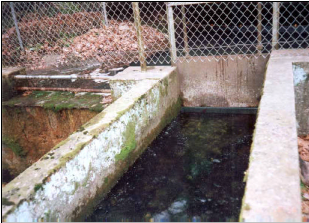
Figure 3. Sluice leading to waterwheel at the mouth of Cave Springs Cave during base flow (stage < 10.98 ft.). Note that there is no waterfall to the left of the sluice.
