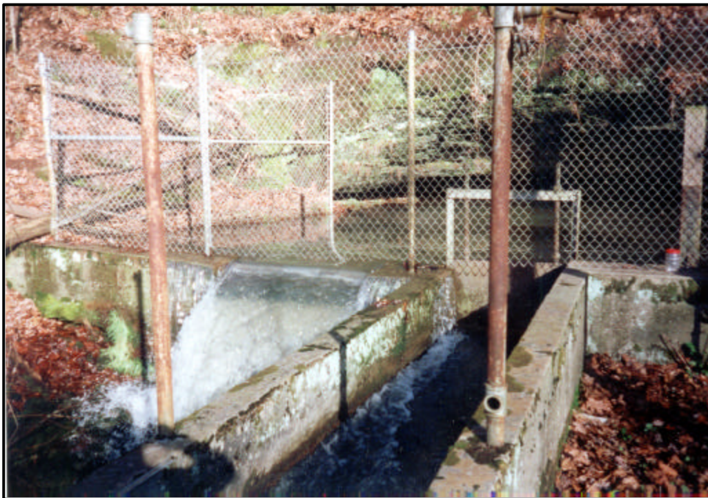
Figure 4. Cave Springs Cave sluice during high flow (stage =12.24 ft.), with a waterfall formed from the overflow channel.
