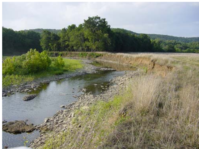
Figure 3. Site 5 – Bank destabilization and erosion
