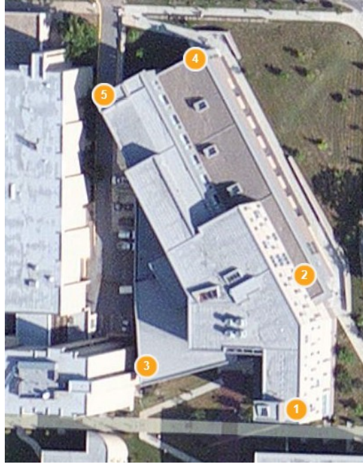
Figure 8. Indoor Testing Area [17].
