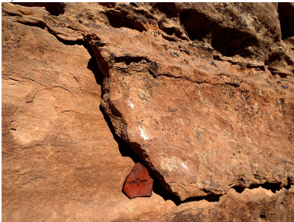
A.34: Large spall preparing to detach on the eastern face of Djinn Block X. Photograph by K. Groom (2013).
