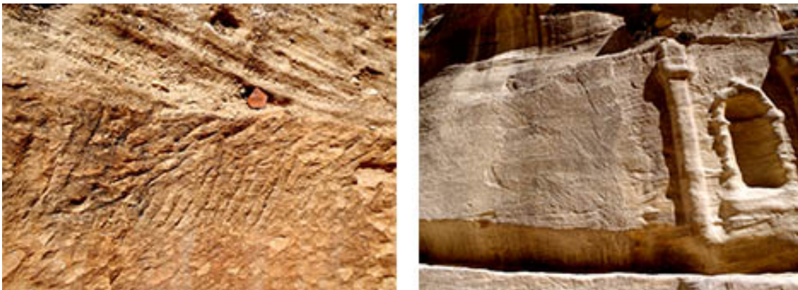
Figure 2.9 – Examples of Nabatean stone dressings: Close up of herringbone dressing on Djinn Block X (left) and a large dressed surface near the opening of the Siq (right). Photographs by K. Groom (2013).
