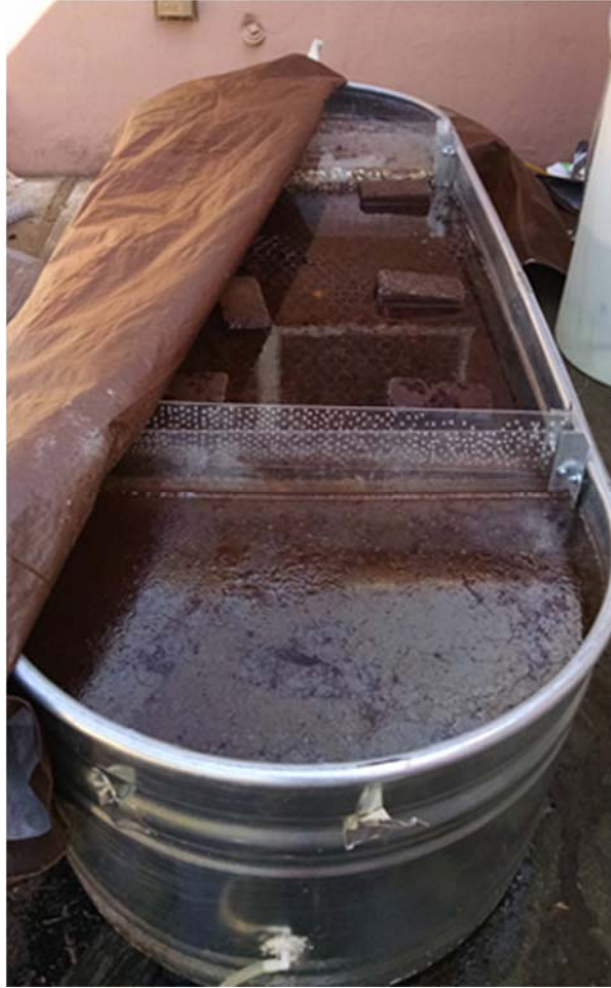
Figure 17: Photograph of completed denitrification bioreactor.
