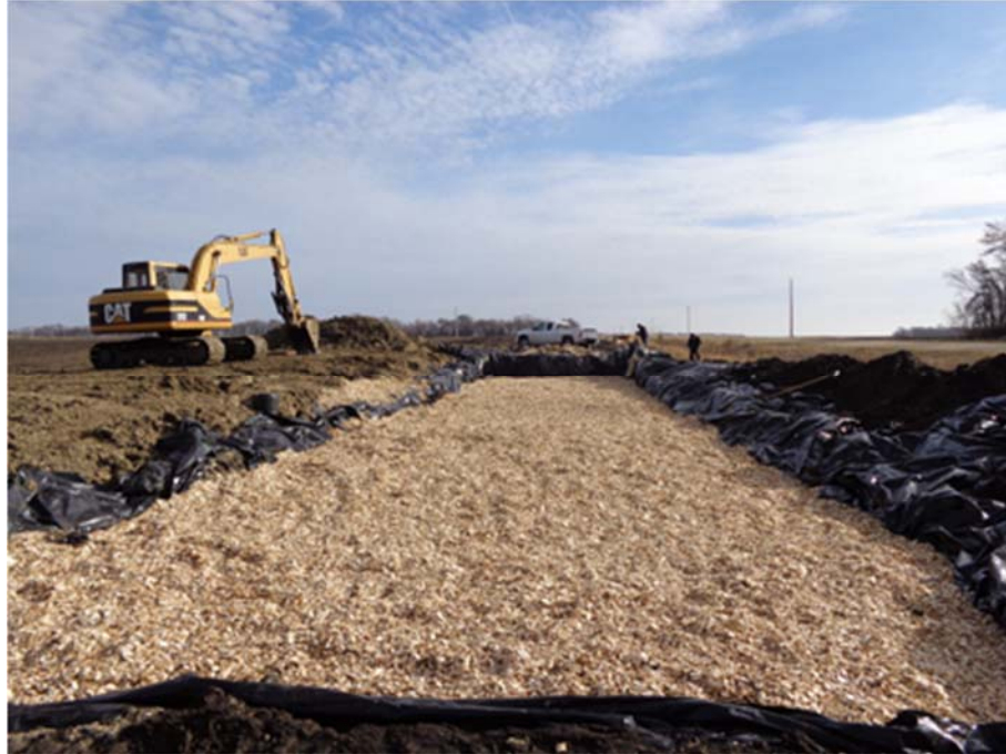
Figure 24: Construction of a large-scale denitrification bioreactor in Iowa (Christianson).
