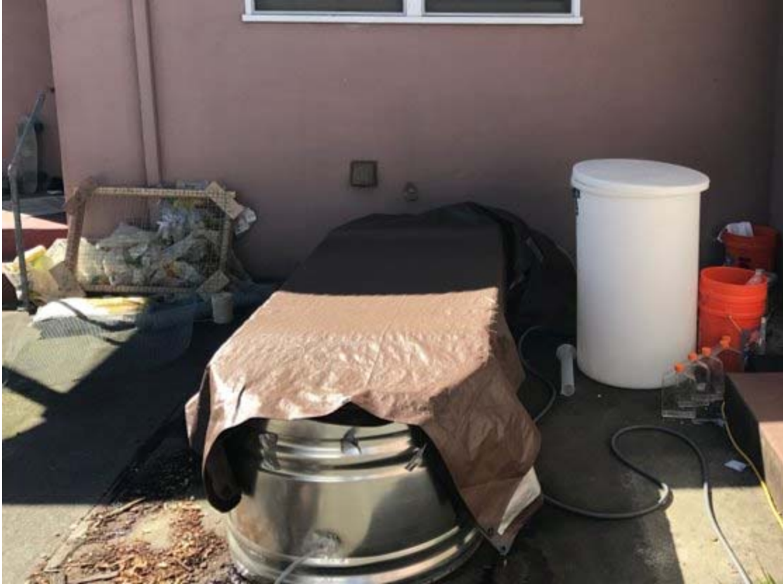
Figure 16: Photograph of completed site setup.
