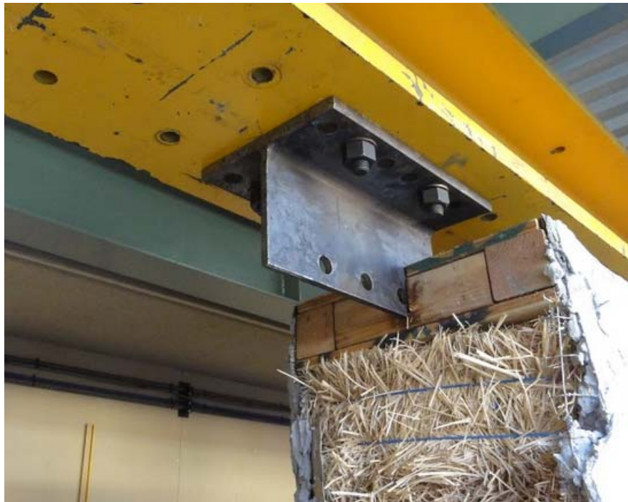
Figure 6: T-Plate slotted into the cap of the Welded-18 wall.
