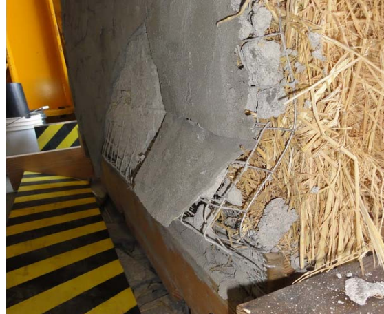
Figure 11: Wire mesh buckling at the base of the wall near the end of the lateral test, after peak displacement had been reached. Each side was repetitively subjected to compression and then tension.
