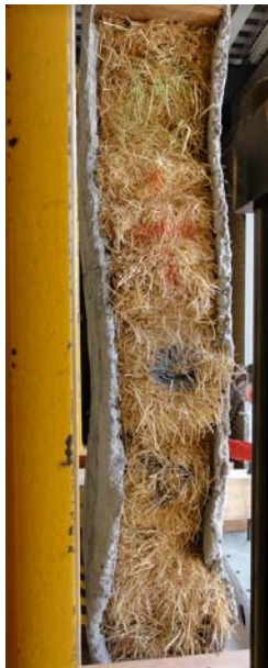
Figure 22: A picture of the Welded-14 wall prior to testing. The wall was not uniform and bore a distinct vertical warp.
