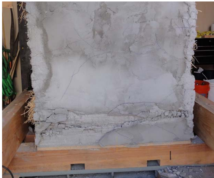
Figure 24: Damage at the base of the Welded-14 wall post-lateral test was concentrated approximately 10” above the base of the wall, due to the extra 10” band of wire added to the modified workhorse connection detail. The outer layer of plaster delaminated from the left side, but the inner layer remained intact, protecting the staples underneath.
