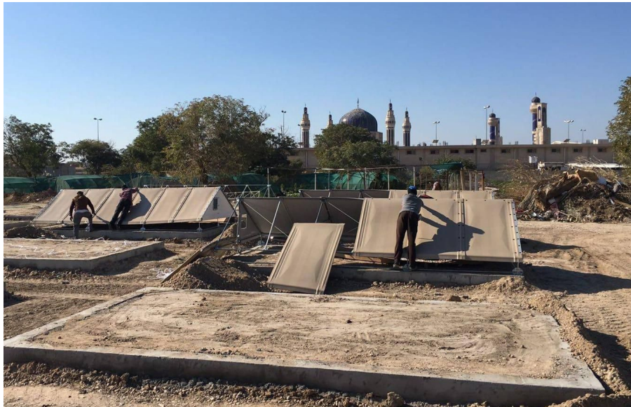
Figure 43. Better Shelters under construction in Iraq.
