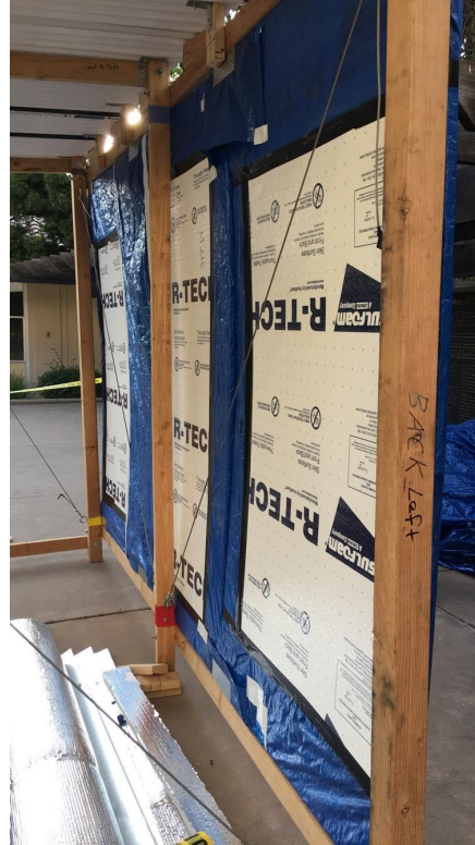
Figure 35. Typical Wall: Connection & Insulation
