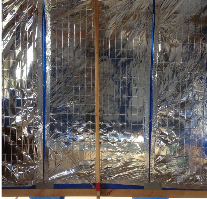
Figure 37. Typical Wall: Inside View with Insulation
