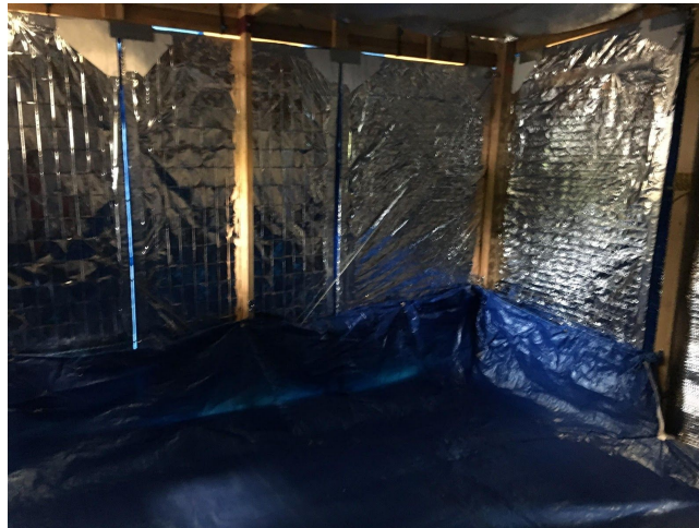
Figure 8. Tarp & Insulation Floor Inside View.
