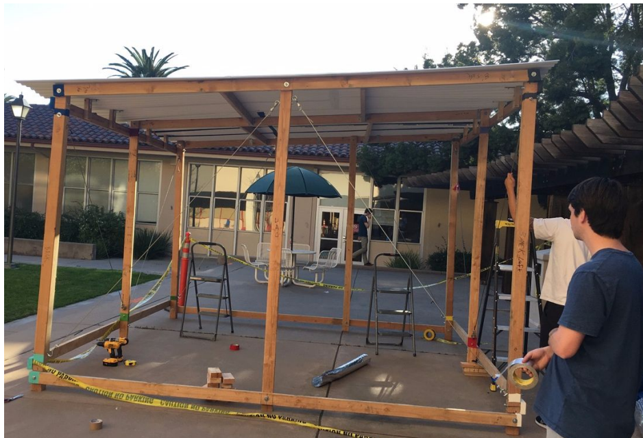
Figure 30. Roof and Frame: Finished framing with completed roof
