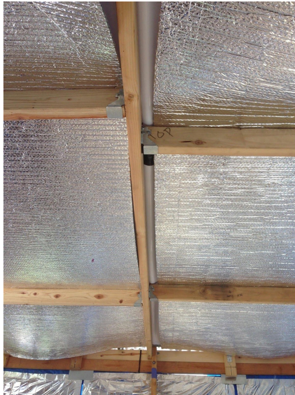
Figure 5. Inside view of roof with insulation.
