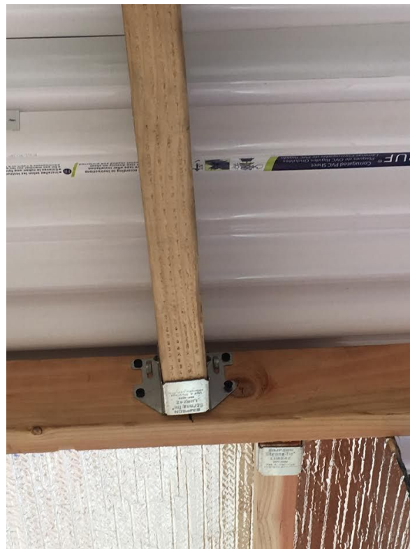
Figure 34. Roof Cross Bracing: Typical connection
