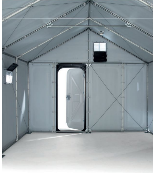
Figure 42. Steel framing system with steel tension cables.
