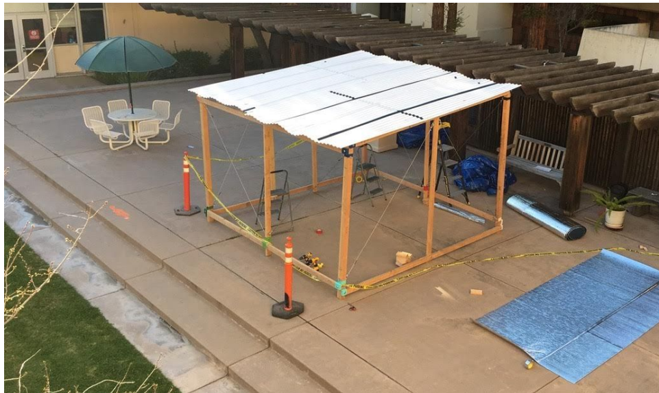
Figure 4. Corrugated PVC Panels bolted on to the shelter structure.
