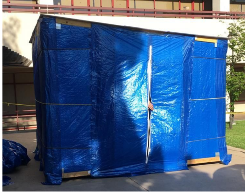
Figure 9. Door Outside View.
