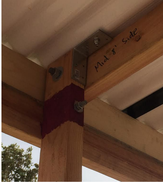
Figure 33. Frame to Roof: Midsection connection
