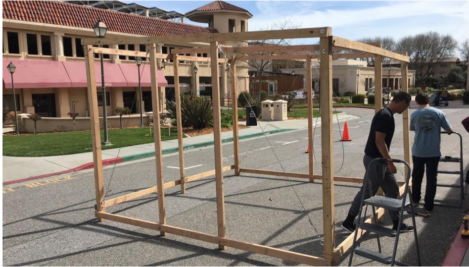
Figure 3. Shelter Structure frame, showing the bolted connections and tension cables.
