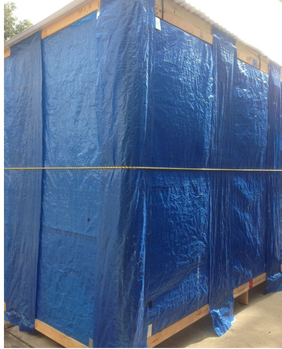
Figure 6. Typical Wall Panel Outside View.
