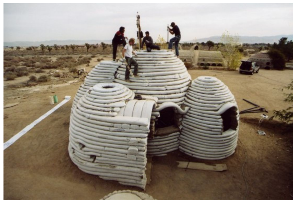
Figure 47. Shelter Sandbag Arrangements.
