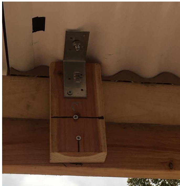
Figure 32. Frame to Roof: Typical connection
