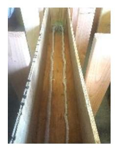
Figure 9: Fish netting rod set into the formwork.
