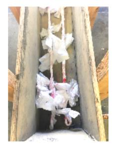
Figure 8: The plastic grocery bag rods set into the formwork.
