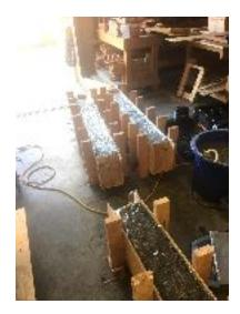
**Figure 10: Poured concrete beams sitting in the formwork.**
