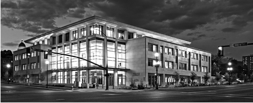
Fig. 15: The Church History Library building, Salt Lake City. © R. J. Olsen, C. McAfee.
