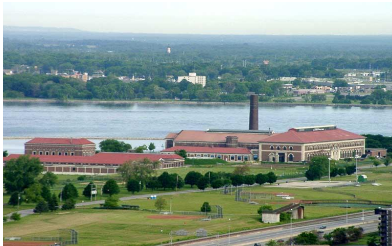
Colonel Ward Pumping Station on Porter Ave. 1
