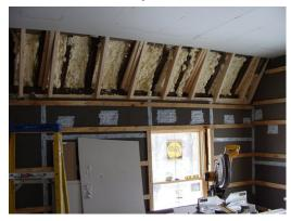
Zero house not only to use clean energy, but to use energy more efficiently. With this concept in mind, PUSH Buffalo created a "thermal envelope", insulating the house with three different types of insulation. They first installed rigid foam board over the studs of the house; then they had dense pack cellulose blown into the spaces between the foam board and the studs. Finally, they used spray foam insulation was to insulate any small cracks that might allow energy to escape.
