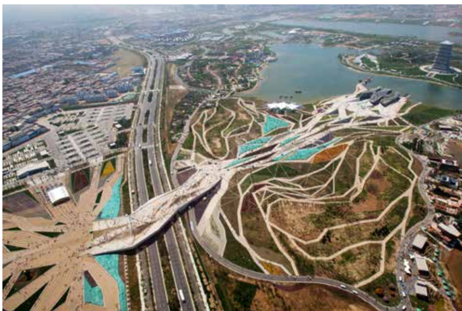
▲ Plasma Studio + Groundlab, Flowing Garden, Xi'an (foto di Plasma Studio + Huashang Newspaper)
