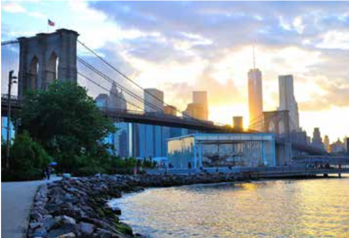
▲ Michael Van Valkenburgh Associates, Brooklyn Park Bridge, New York, 2003-2016 (foto di dumbonyc)
