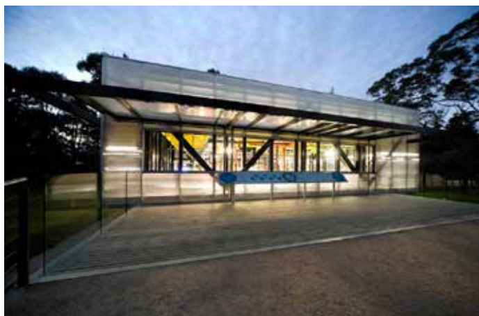
▲ Peter Elliott, Zoo Water Treatment Facility, Melbourne, Australia, 2007 (foto di John Gollings)
