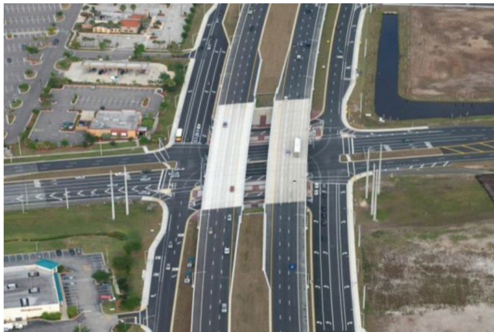
Figure 2.3 Tight diamond interchange.
