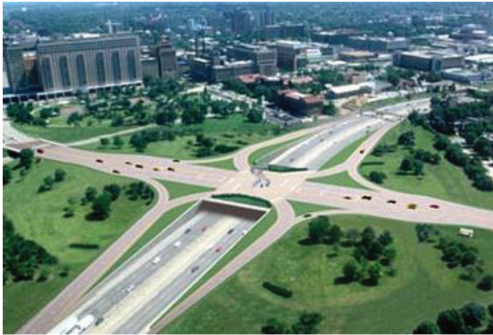
Figure 2.4 Single point interchange.
