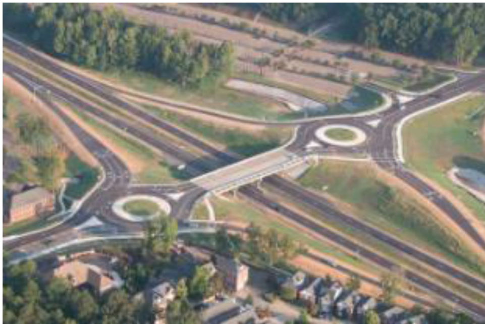
Figure 2.5 Double roundabout diamond interchange.
