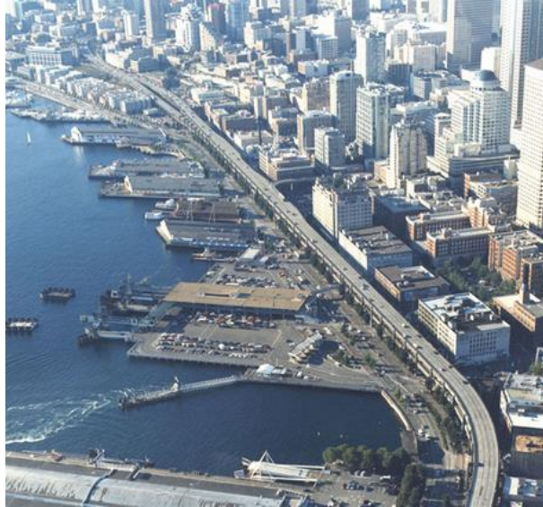
Figure 6.1 The Alaskan Highway Viaduct has acted as a major thoroughfare moving Seattlites from one end of the city to the other for fifty years. Although it will be torn down and replaced with an underground passageway, its path will mimic the viaduct in order to link to the city's current infrastructure.
