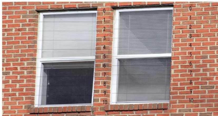
Figure 3.1. Window on left has 60% occlusion from blinds with slats closed, whereas window on the right has its blinds 100% closed, with slats open.
