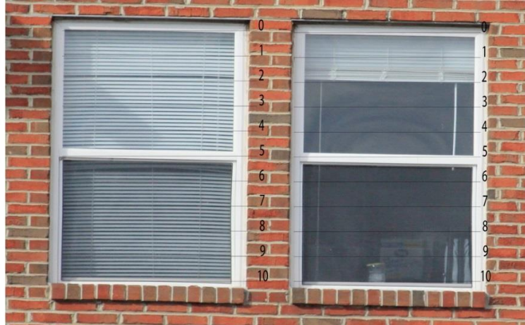
Figure 3.2. Left side window has 100% occlusion whereas window on the right has 20% occlusion.
