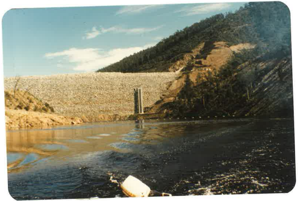
Fig. 5.5 : Dartmouth Dam, Mitta Mitta River. View west from site 2 to site 1, just upstream of the retaining wall.
