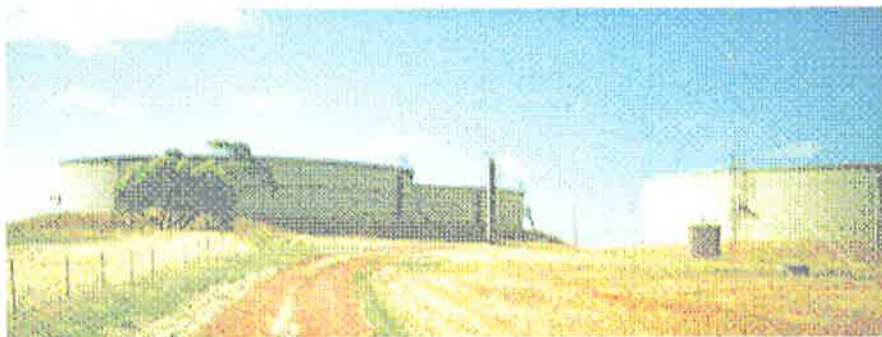
Figure G.4 Arthurton Tanks
