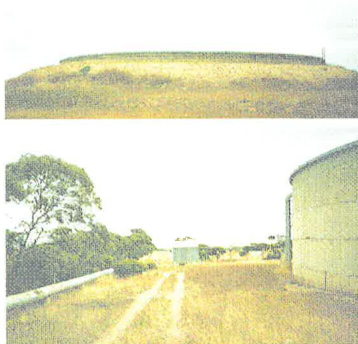
Figure G.2 Maitland Tanks
