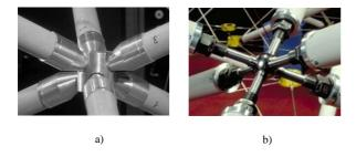
Figure 3: Two stages of the central joint development: (a) three module structure central joint (Fest et al. 2003) and (b) five module structure central joint
