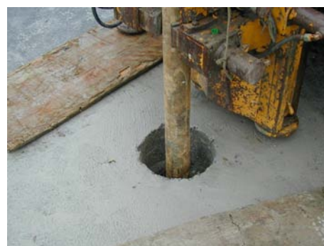
2m depth drillhole
