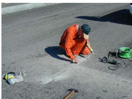
Temperature probes located at the HMF – HMT interface (-12cm). Probes were fitted with silicon.
