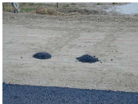
Temperature probes PT100 at -26cm. Left: detail of the probe. Right: HMF laying. Probes were protected with a fine bituminous layer.
