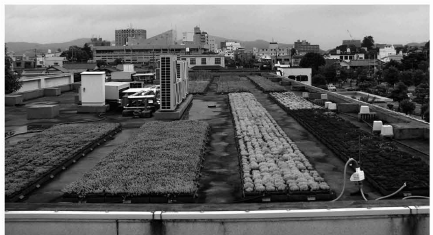
Fig. 1 Roof-top view of Kanrito-building (Research Institute for Bioresources) in June, 2008. Sedum species were planted over the thin-layer/Excel soil© system.
