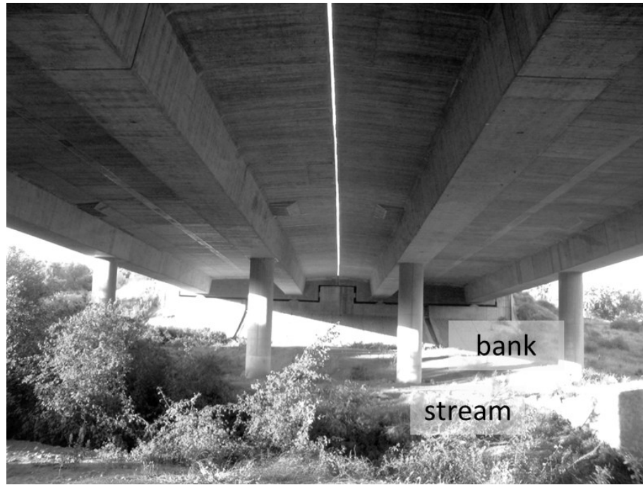
Fig 6.5 – Example of an eco-passage in A6: an extended stream crossing. Vegetation at the entrance and along the passages could be planted to minimize human presence and favor animal use. Large banks provide best conditions for animal use.
