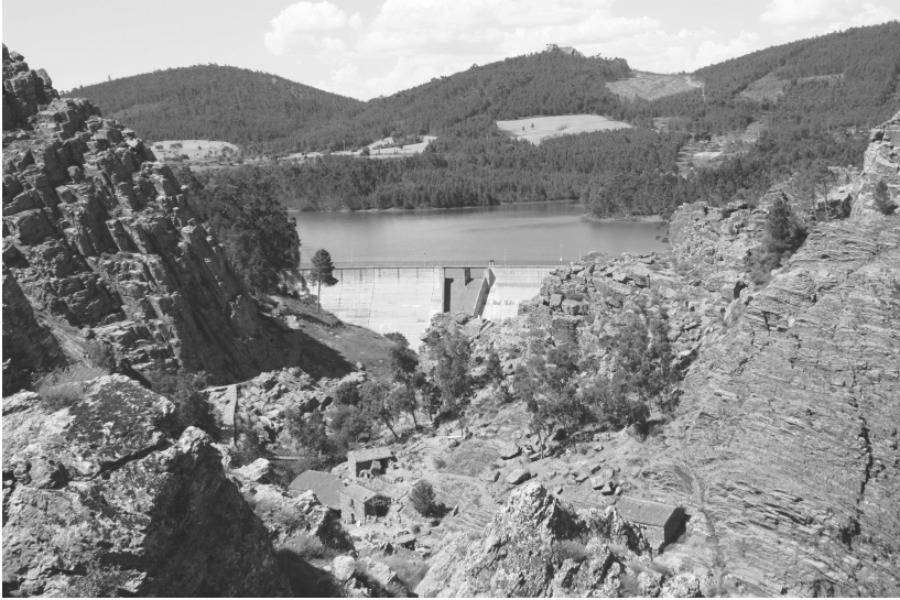
FIGURE 13.3. Penha Garcia Dam, concluded in 1979, on a gorge of the Ponsul River (photo by Pedro Pinto).
