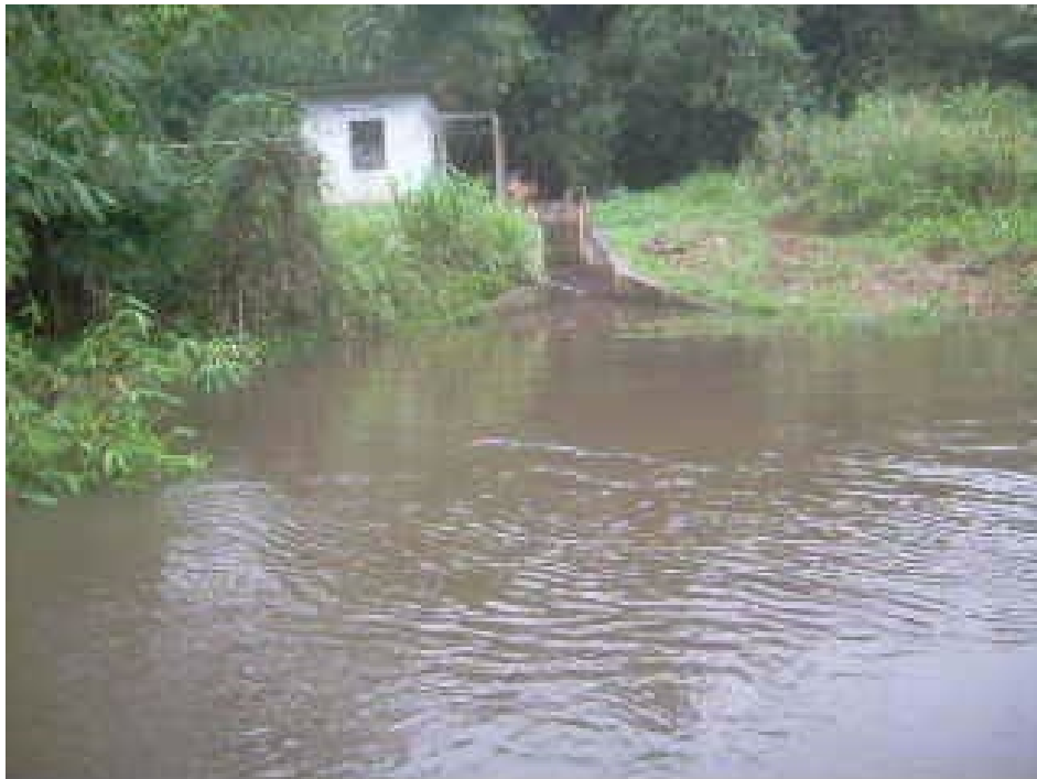
Plate 4.6: Water intake station for Ogun State Water Corporation
