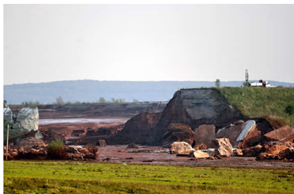
Image 2: Kolontar (Hungary). Failure of the ‘red mud’ dam retaining wall, 12 October, 2010. .
