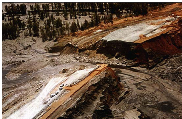
Image 1: Aznalcollar (Spain). Failure of tailings dam retaining wall, 25 April, 1998.
