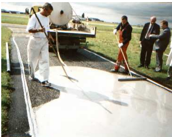
Figure 2. Cementitious slurry grouting on the hot mix hot laid porous asphalt.
