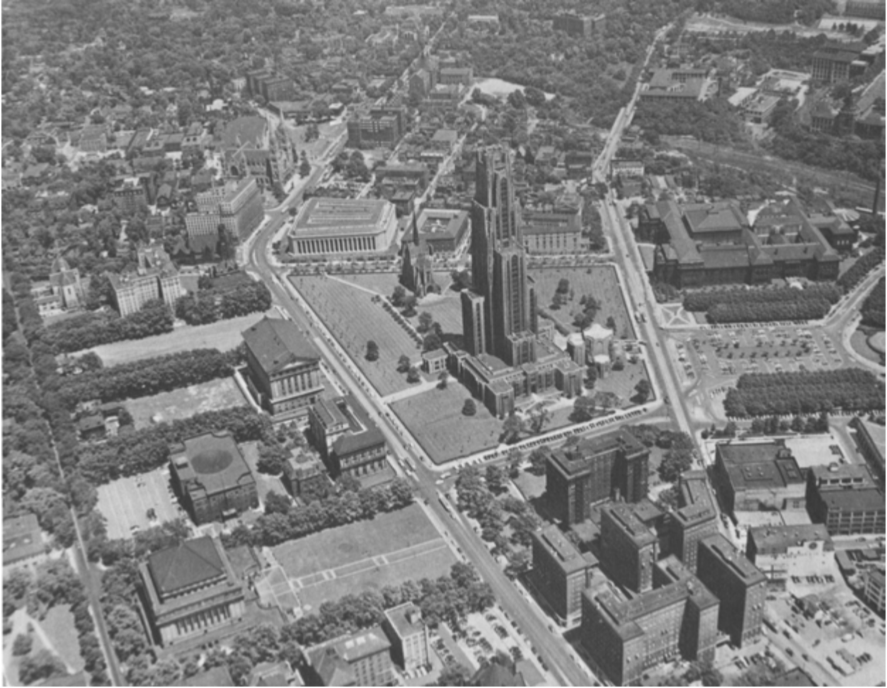
Figure 2-20: Oakland. Pittsburgh Regional Planning Association. A Plan for Pittsburgh's Cultural District, Oakland (Pittsburgh: Pittsburgh Regional Planning Association, 1961), inside front cover. University of Pittsburgh, Hillman Library.
